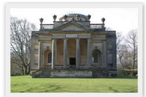
Above: Gibside Chapel
